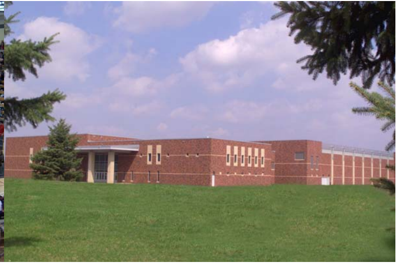
Exterior of Building
